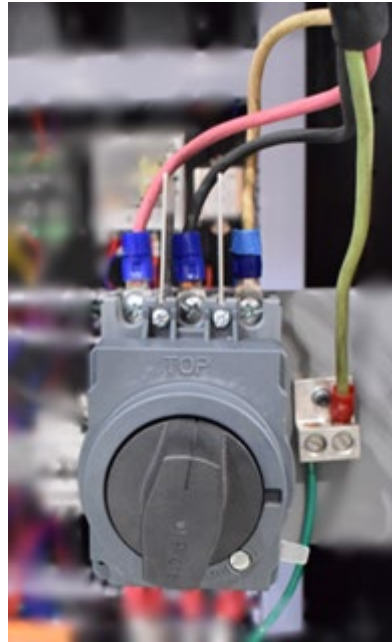
Figure 5-2: Main Disconnect and Ground Lug (3-Phase)
